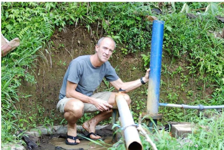
property and pay between 6000 and 15000 rupiah a month based on the meter reading towards maintenance of the system. But pumping the water from the spring to the collection tanks in the village, 850m away and 56m higher, isn't an easy task. With no electricity anywhere nearby a gravity pump, using water to pump water, is one of the few options available. Although a gravity pump is of a simple construction with few moving parts and is often used in rural
